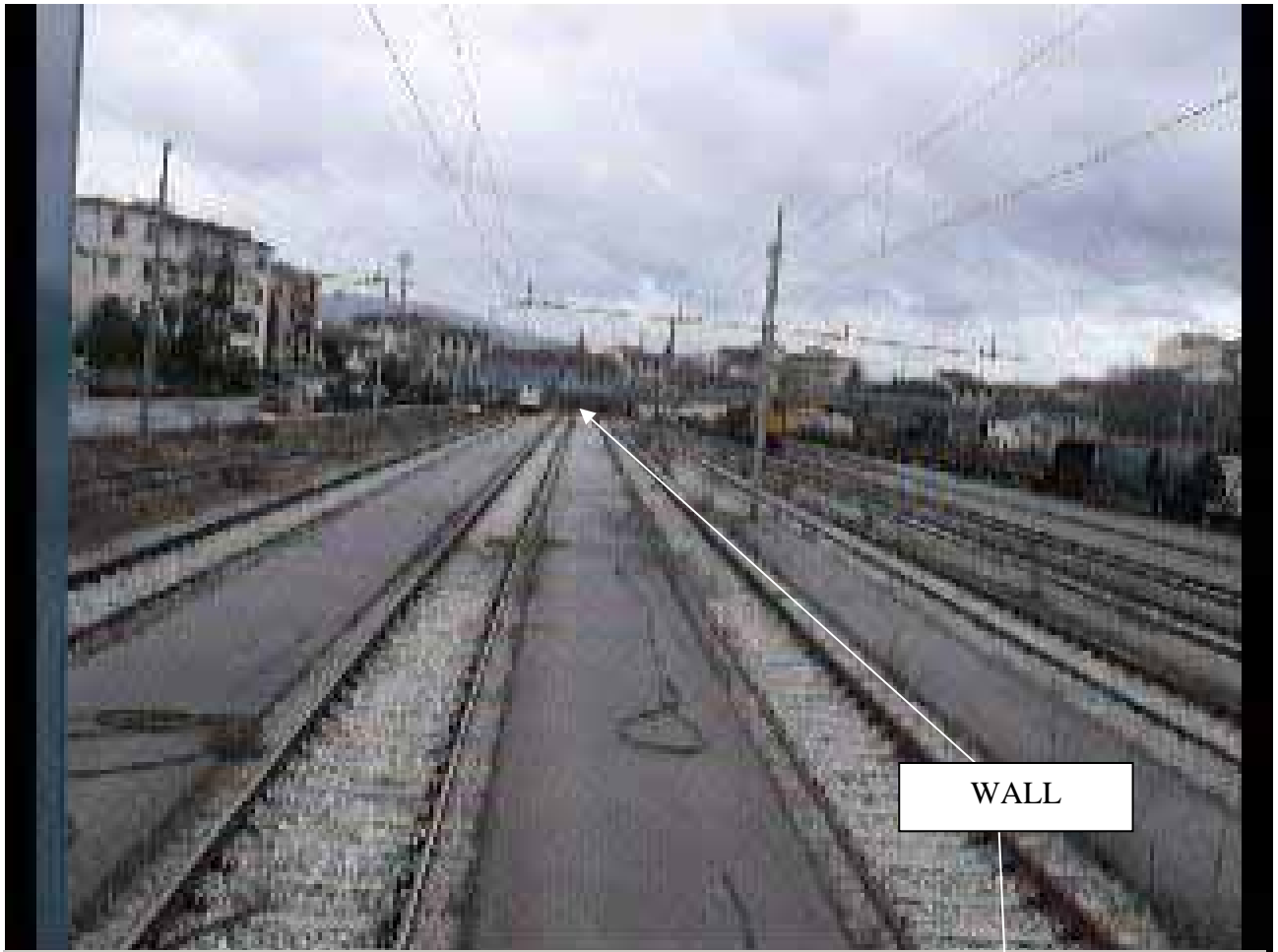
The wall at 234m.
