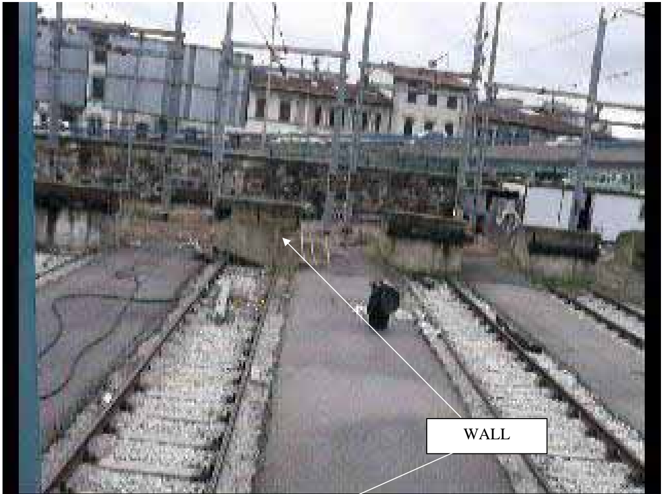
The wall at 24m.
